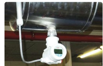
VortexMaster installed in an insulated steam pipe
